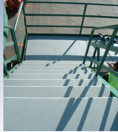
Boarding stairway with smooth anti-skid surface and integrated heating function.
