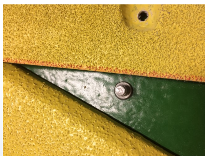
Deck fastening detail (Hilti X-BT)
